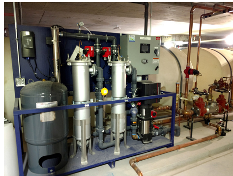
UV System Installation
