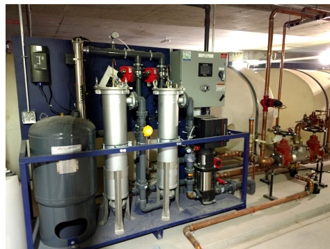
UV System Installation
