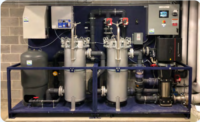
UV System Installation
