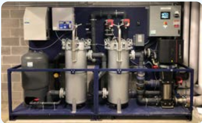
Ozone System Installation
